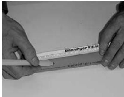
Fig. 5 Mark out the socket depth.
