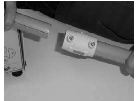
Fig. 6 Push in the socket up to the marked position on the pipe.
