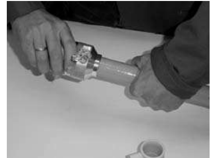
Fig. 3 On Bänninger Stabi-Pipes , the aluminum coating must be peeled off before jointing.
