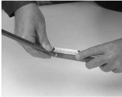
2. Clean the joint area with cleaner. Mark the insert depth of the fitting on the pipe.
