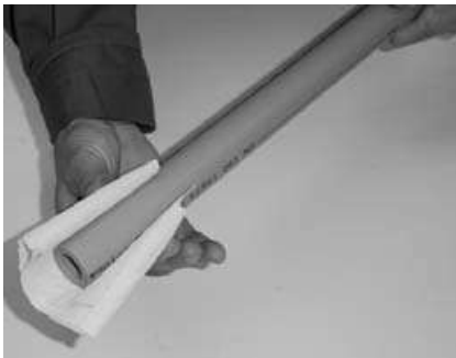
Fig. 4 Clean the joint surfaces with a purifying agent (e. g. spirit).
